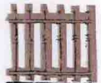
Painted metal railing.
