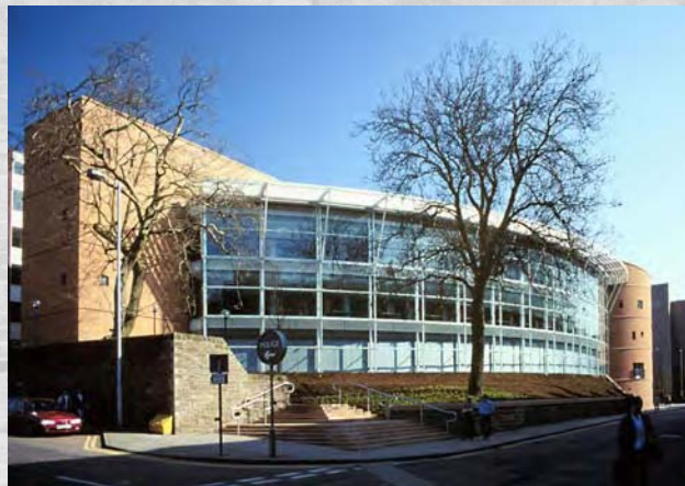
The glass facade of the University of Abertay Library uses the solar gain of a southerly aspect to induce air circulation by natural convection throughout the building. The library continues the set piece design ethos of the Victorian buildings in the area.
