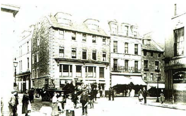
Overgate/Tally Street; late 19th century view. A backdrop of modest mixed use structures formed the counterfoil to the classical public buildings and contributed to a lively streetscape.
