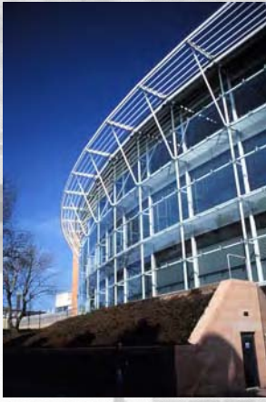
The glass facade of the University of Abertay Library uses the solar gain of a southerly aspect to induce air circulation by natural convection throughout the building. The library continues the set piece design ethos of the Victorian buildings in the area.
