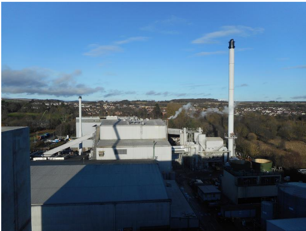
Figure 4 – Site Photo of new CHP facility
