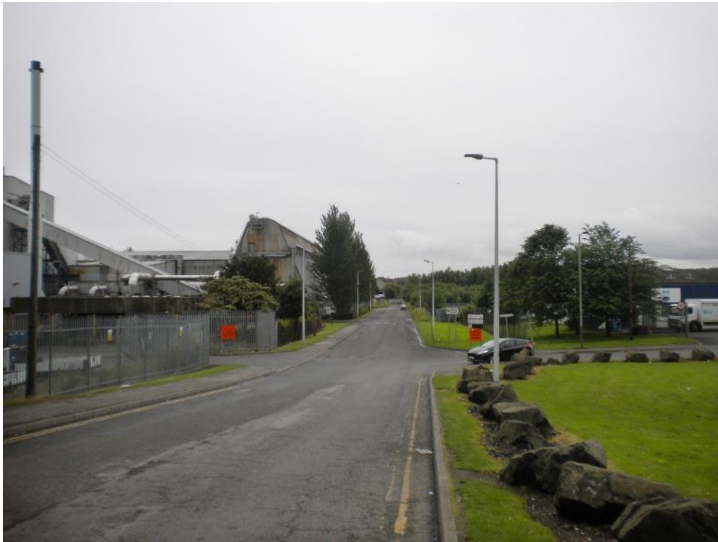
Figure 3 – Site Photo original DERL plant
