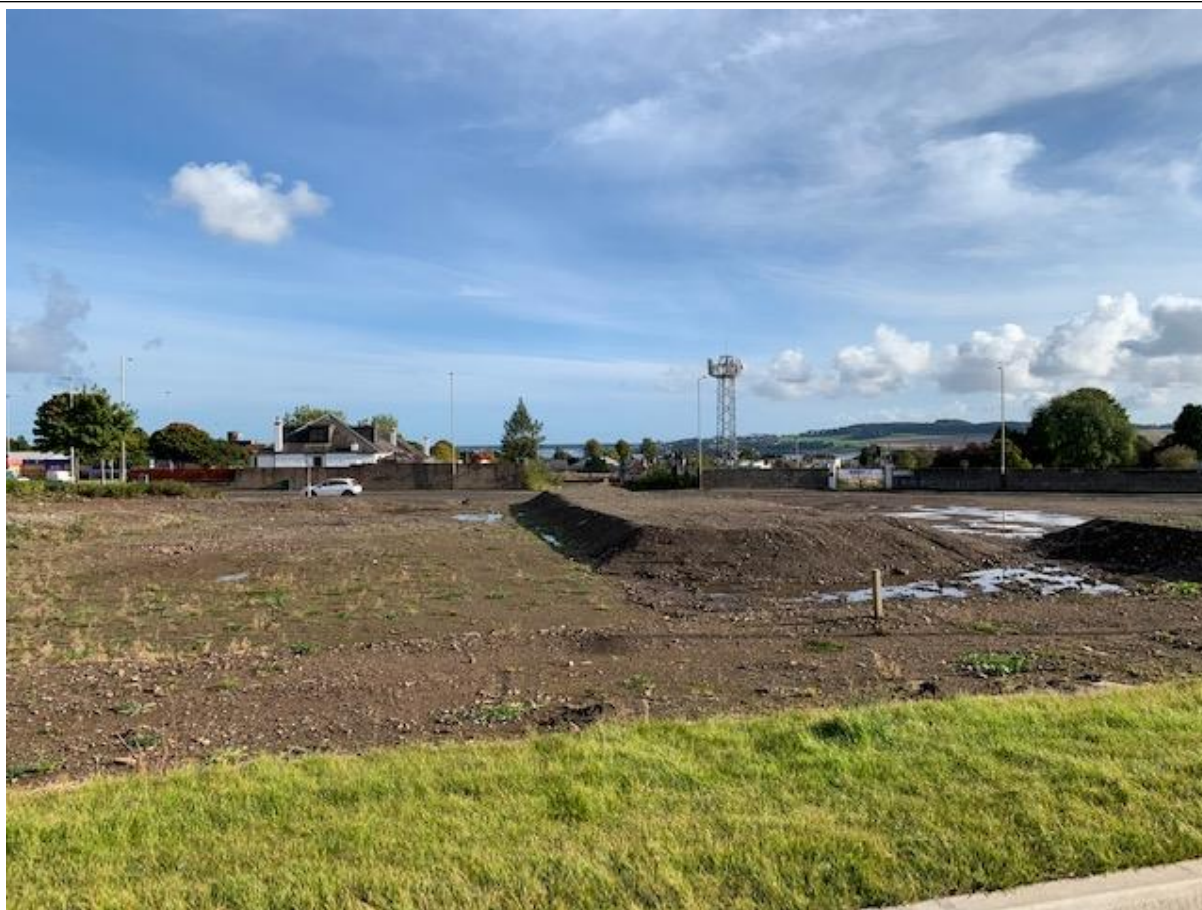
Figure 3 – View Towards Site
