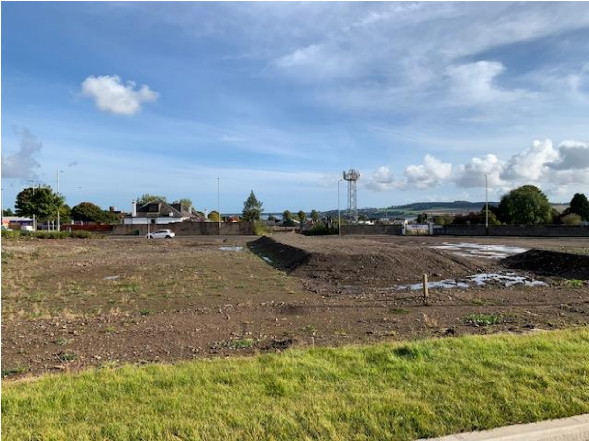
Figure 3 – View Towards Site
