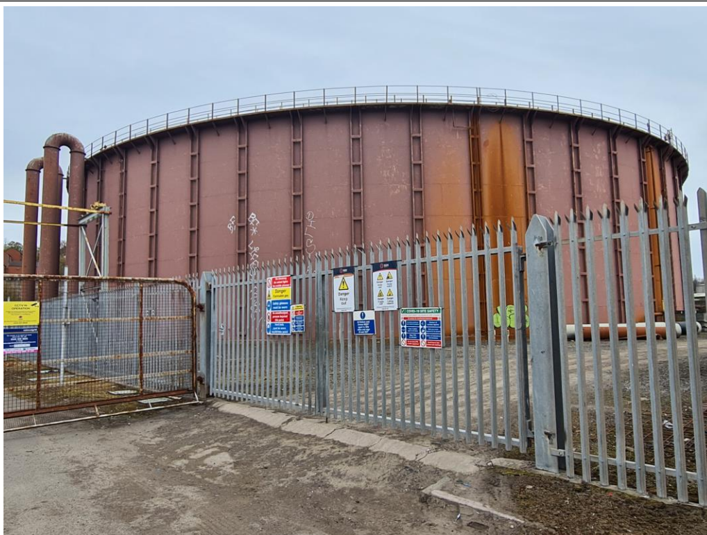
Figure 2 – Photo of site
