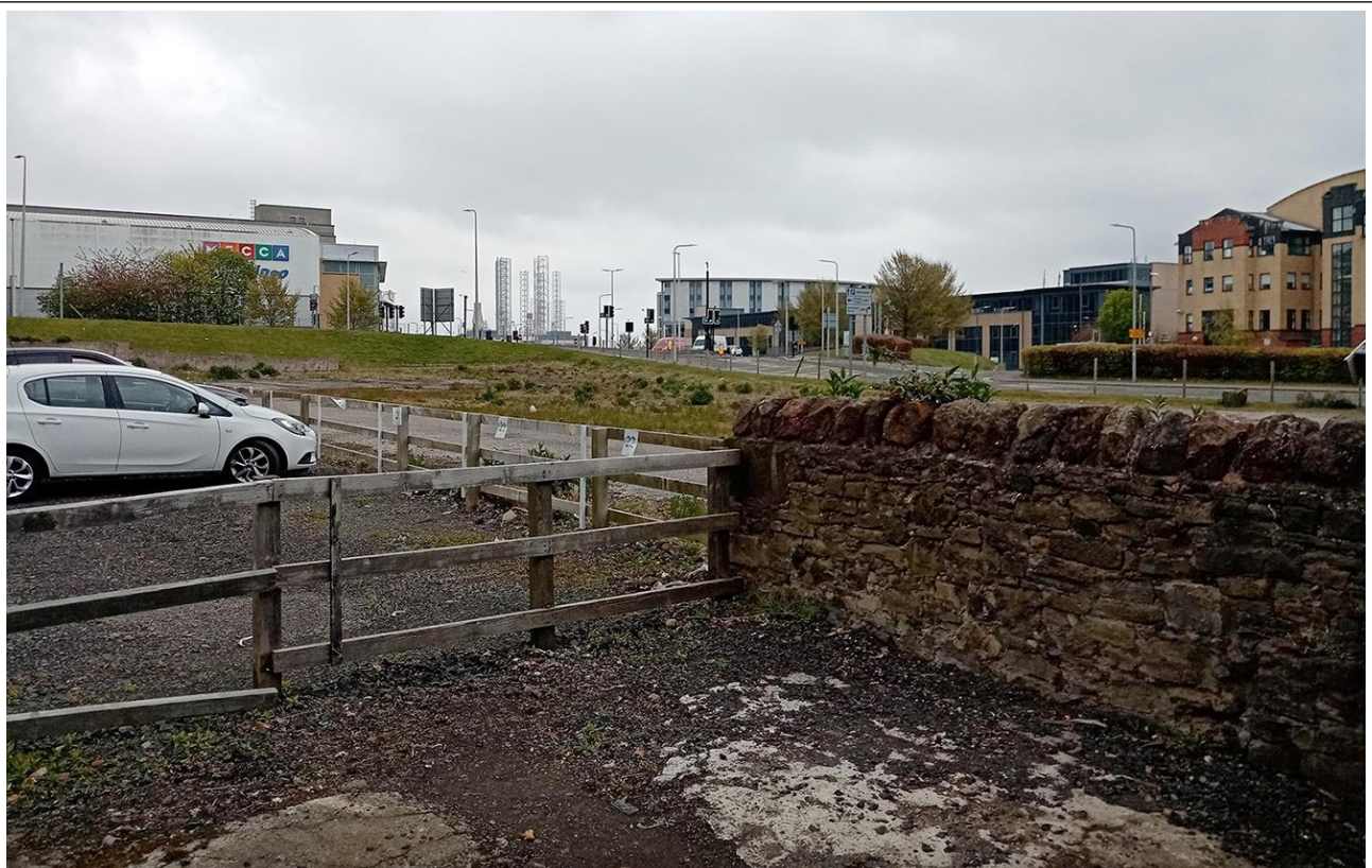
Figure 8 – Remnant Section of Sea Wall With View Towards The Site's South and East Boundaries
