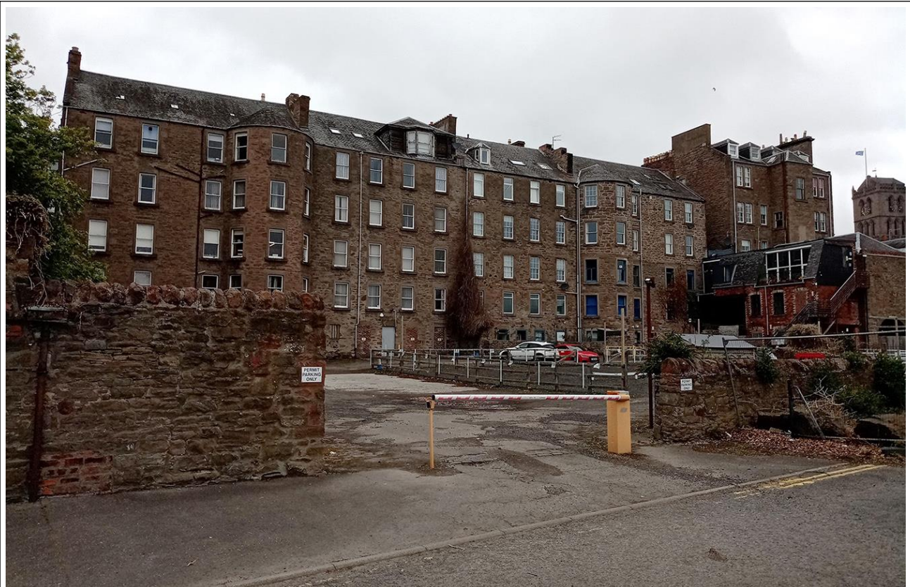
Figure 6 – Rear Elevation of Listed Buildings On Nethergate, To The Site's North Boundary
