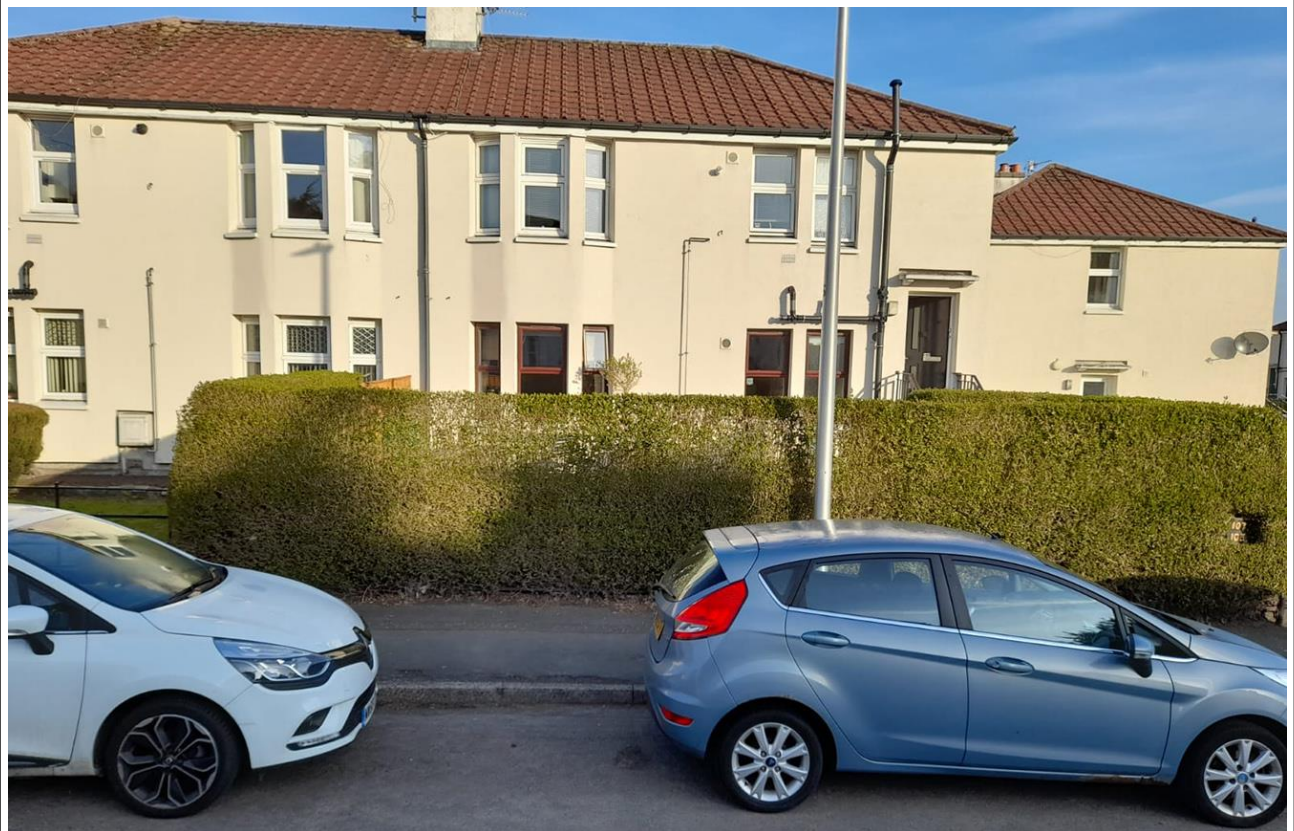
Figure 4 – Photograph of Existing South East Elevation
