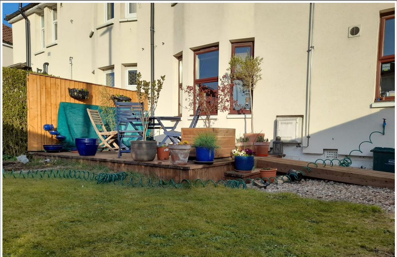
Figure 3 – Photograph of Existing South East Elevation
