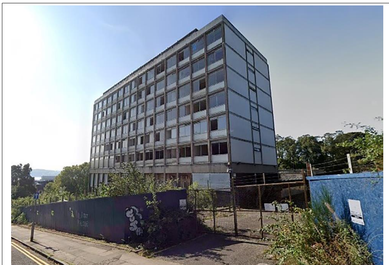
Figure 5 – View of Site from Constitution Road
