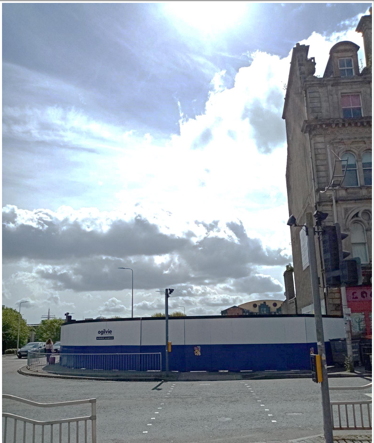
Figure 5 – Application Site Viewed from Nethergate
