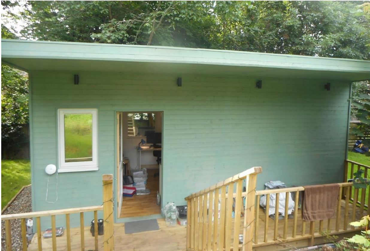
Figure 4 – Timber Cabin A
