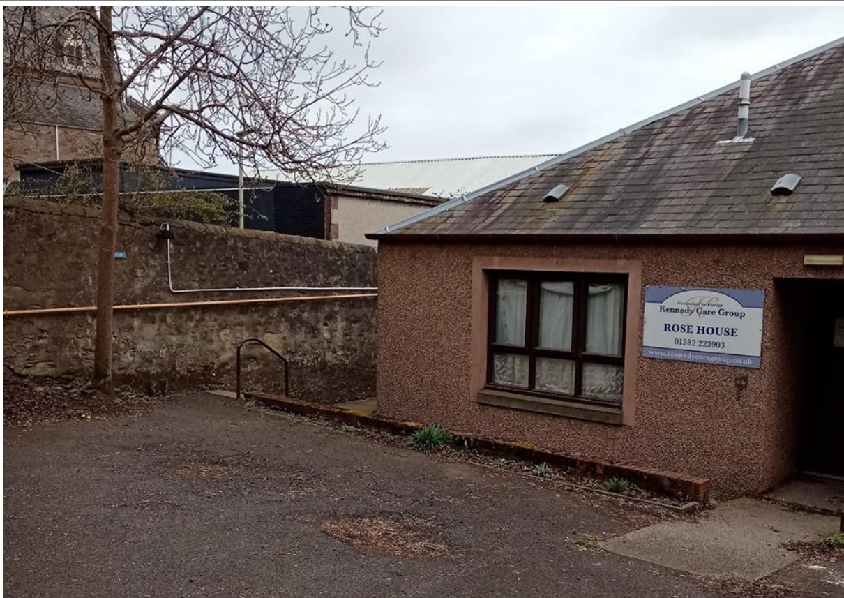
Figure 4 – View of Application Site from Constitution Street (North Entrance)
