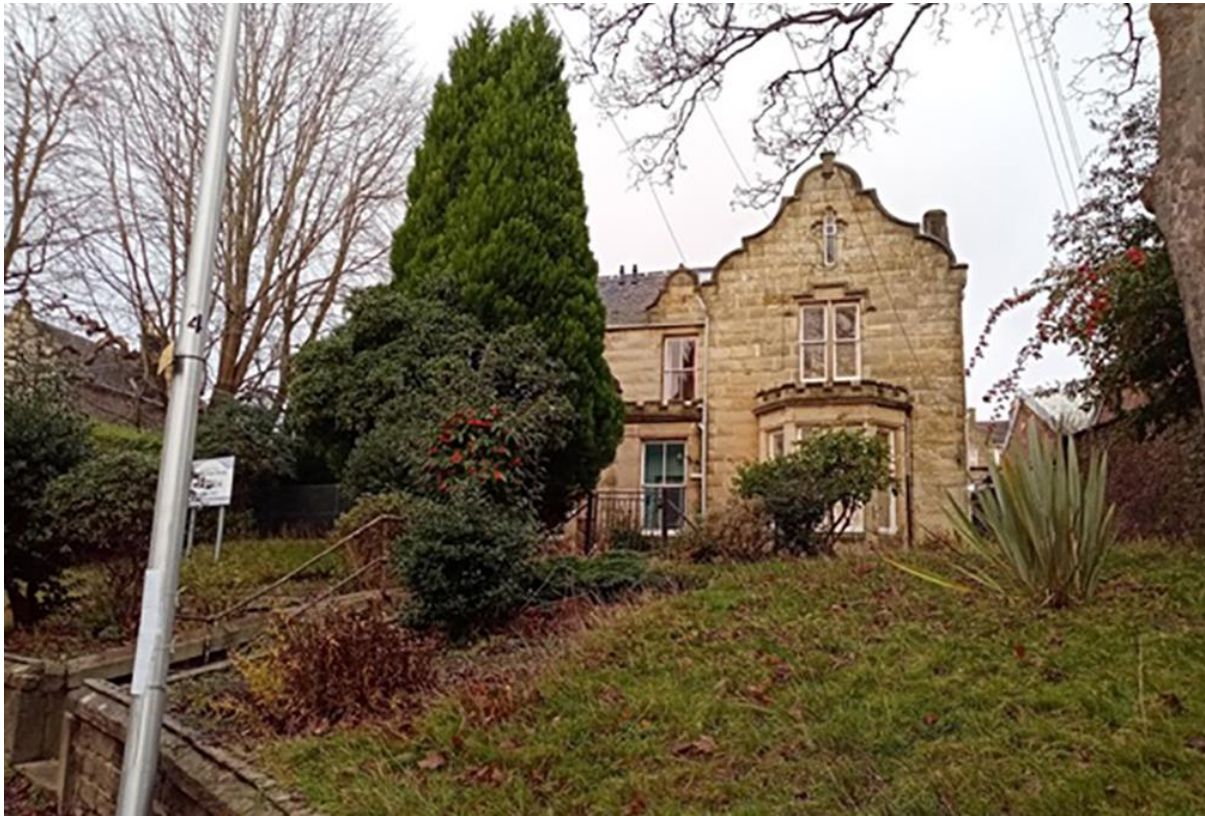
Figure 3 – View of Application Site From Constitution Terrace
