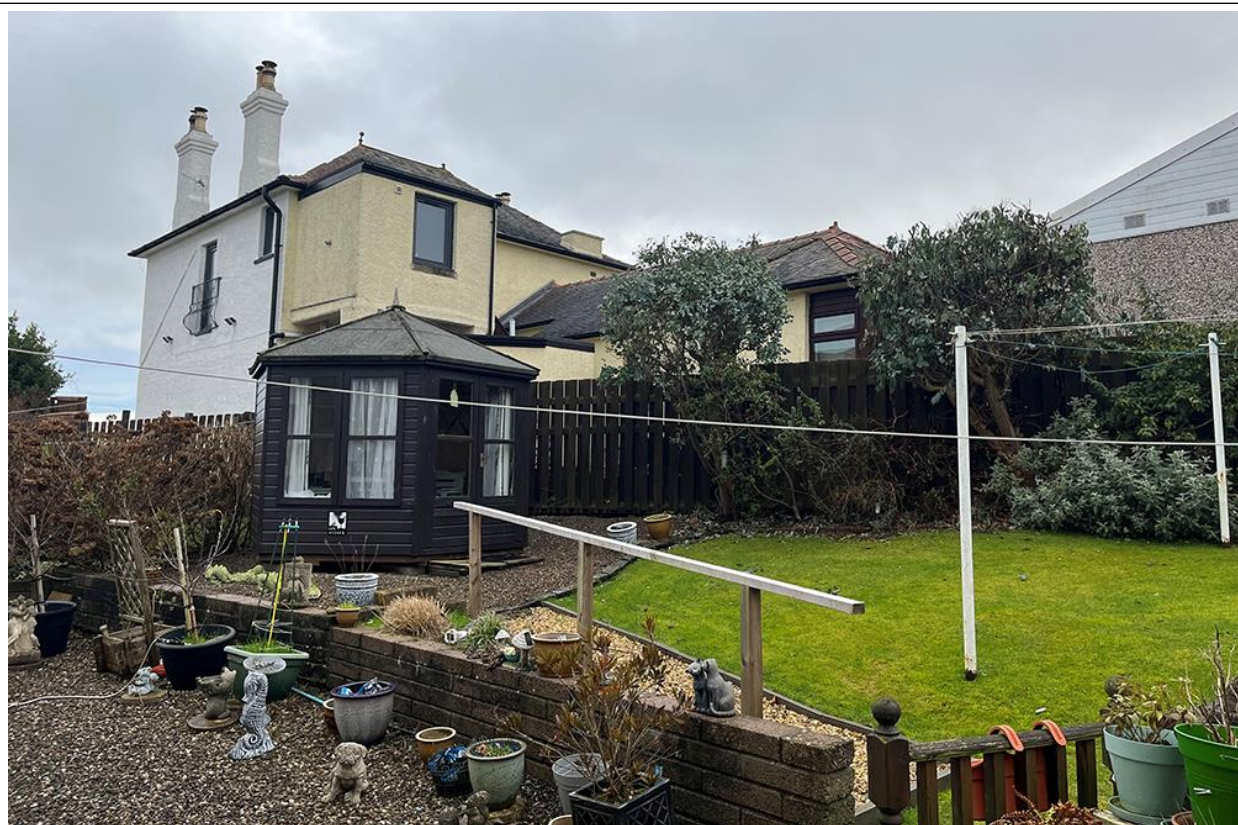
Figure 5 – Photo of Application Dwelling From 39 Broadford Terrace
