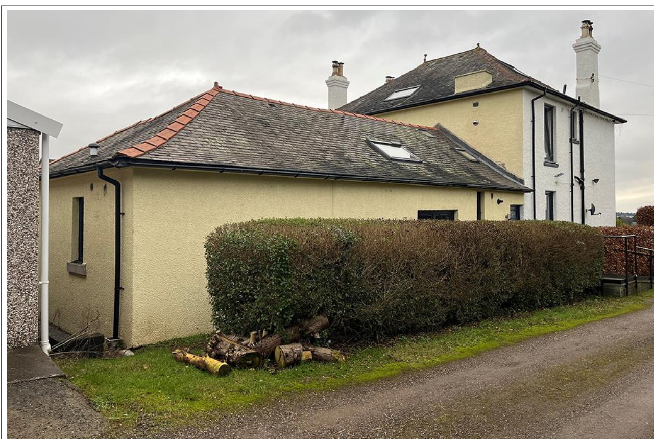
Figure 3 – Photo of Existing Rear Extension From Holly Crescent
