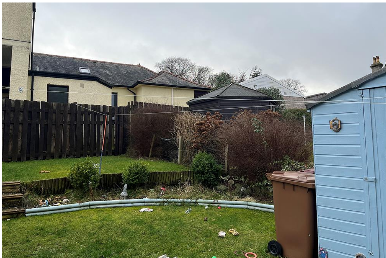
Figure 4 – Photo of Existing Rear Extension From 39 Broadford Terrace
