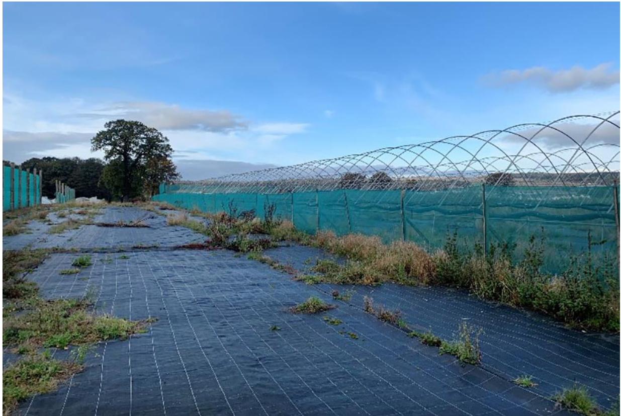
Figure 4 – View of Existing Polytunnels Facing North
