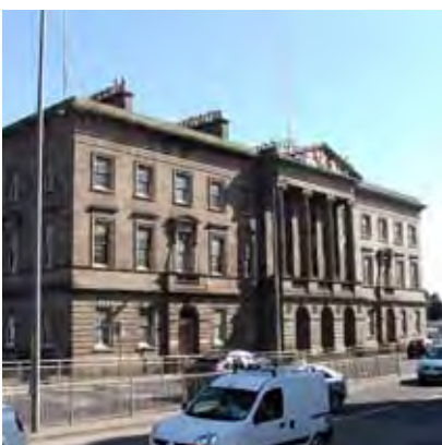
Former Customs House & Harbour Chambers Building
