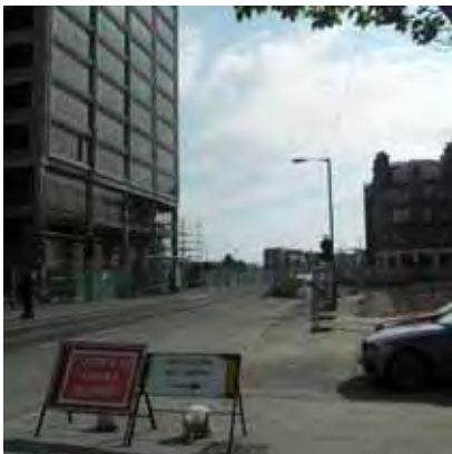
Works underway to demolish Tayside House
