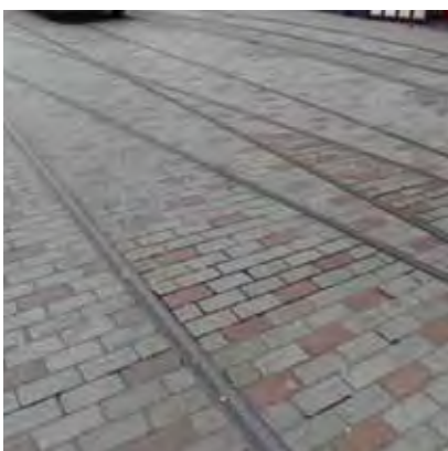
The use of tram tracks as public art within the streetscape
