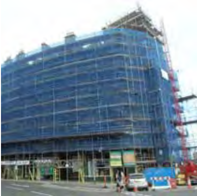
Tay Hotel currently being renovated to become part of the Malmaison hotel chain
