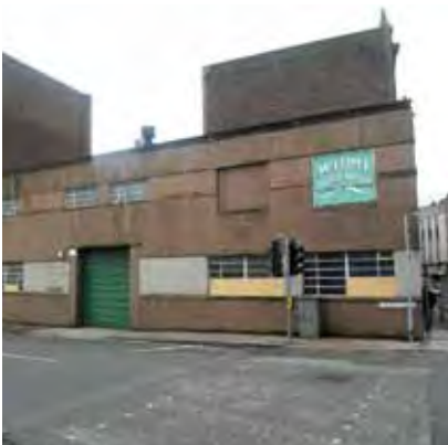
Building in poor state of repair
