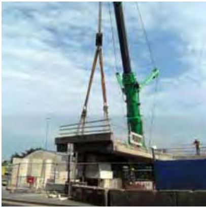
Bridge ramps being reconfigured
