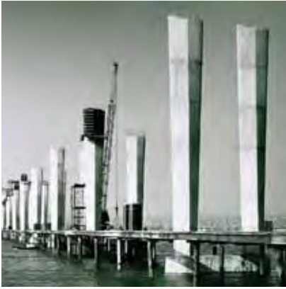
Tay Road Bridge Construction
