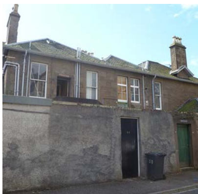
Sensitive wall repair
