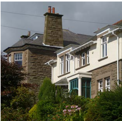
Roof detail and traditional windows
