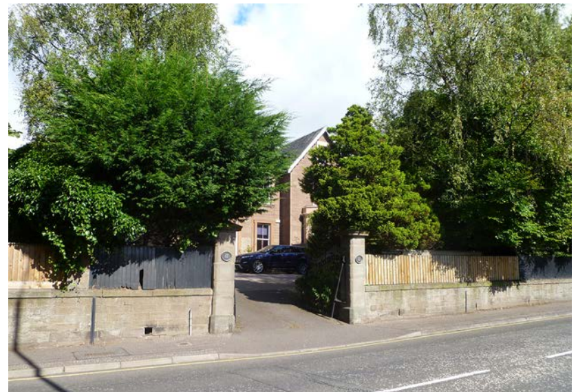
Boundary railings replaced with timber
