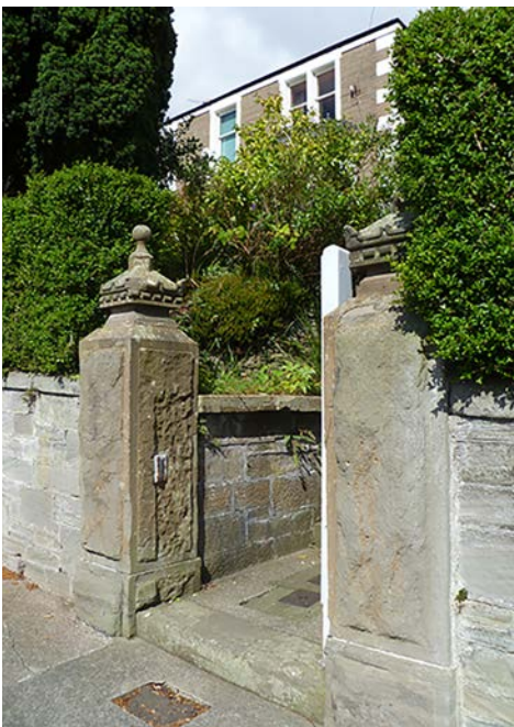
Traditional gate piers
