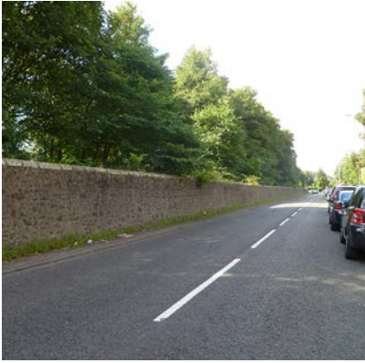
High stone boundary walls and greenery
