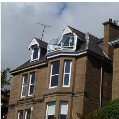
Traditional dormer windows and modern balcony
