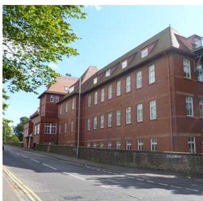
Former Dundee Royal Infirmary building
