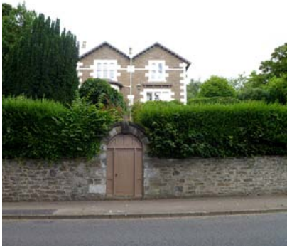
High boundary walls
