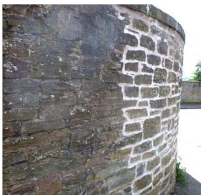
Insensitive wall repairs
