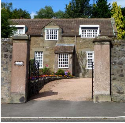
High boundary walls
