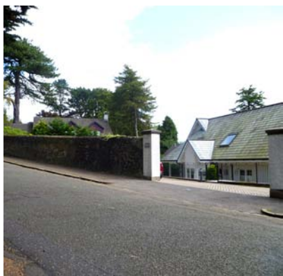
Newer build on Reres Road
