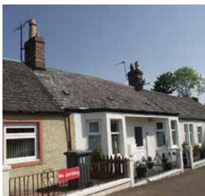
Modern replacement windows
