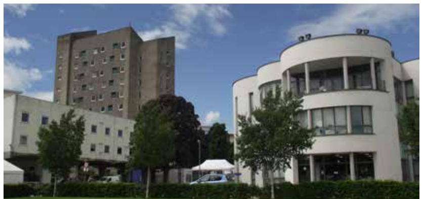
Belmont Towers and the Queen Mother Building
