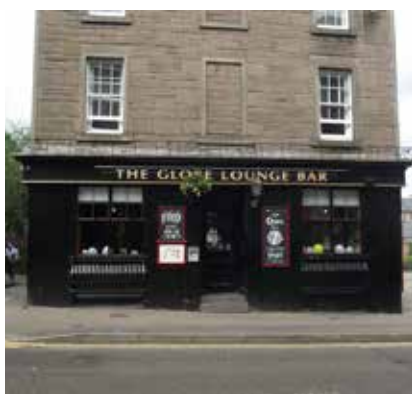
Shop front, West Port
