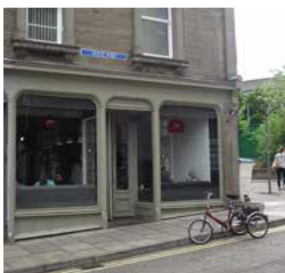
Shop front, West Port
