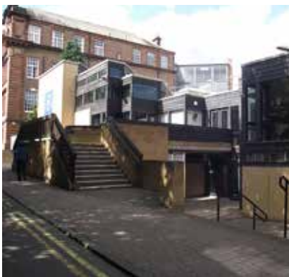
Bonar Hall entrance from Park Place
