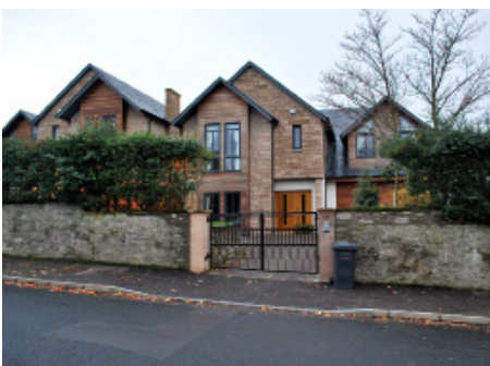
Duntrune Terrace New Build
