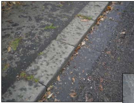
Wide stone kerb with stone drainage channel
