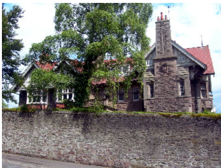
Aystree seen behind high boundary wall
