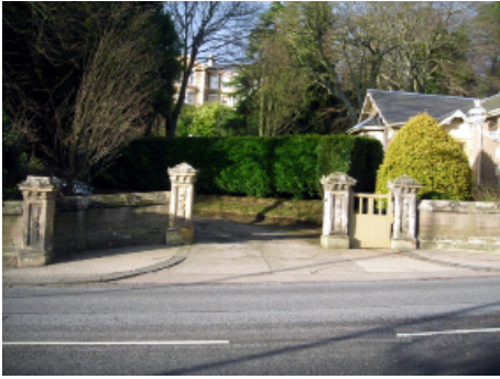
Decorative stone wall and gate piers
