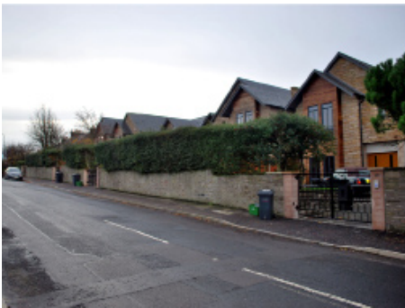
Duntrune Terrace New Build
