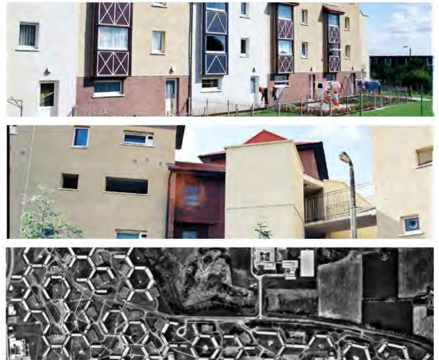
Figure 04: Examples of Whitfield's original housing developments.
