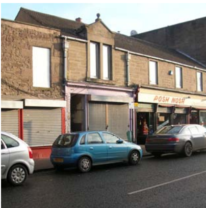
Shutters On Existing Shopfronts
