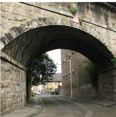
Camperdown Works Railway Bridge
