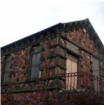
Former Lochee Railway Station
