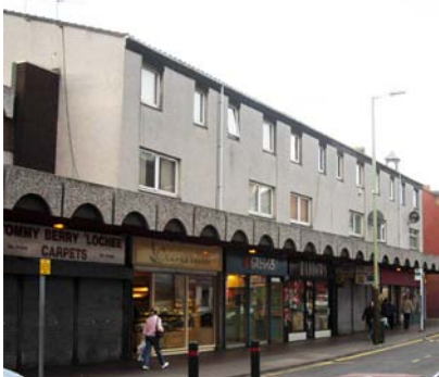
Example of Current Facade
