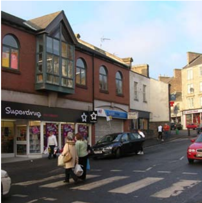
View To North of 139 High St
