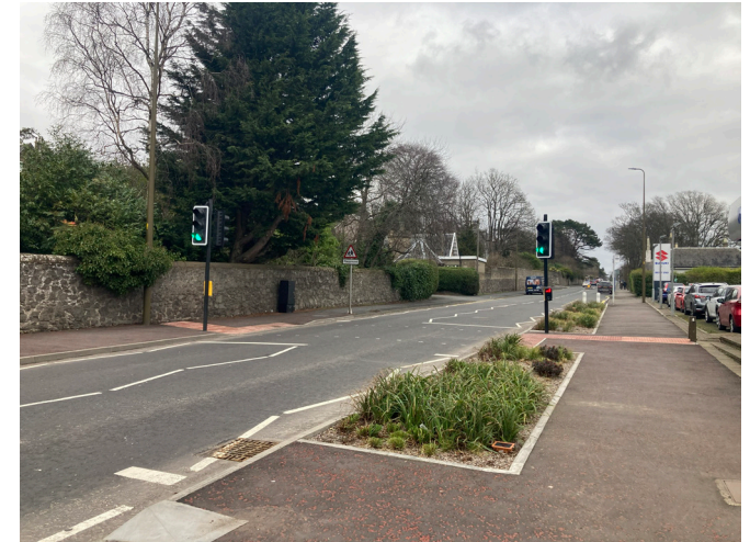
A signal controlled crossing located along Monifieth Road, supported with green infrastructure.
