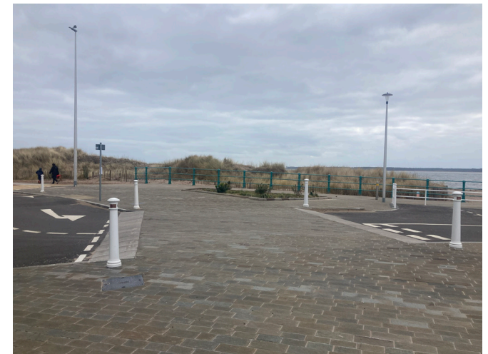
A continuous crossing in Broughty Ferry, located along National Cycle Network Route 1.
