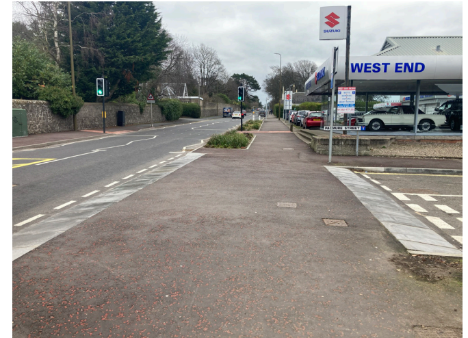
An example of a continuous footway along Monifieth Road.
