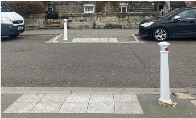
An uncontrolled crossing supported with tactile paving. The crossing distance is reduced by the build-out of the carriageway. Bollards help to prevent vehicle overrunning.
