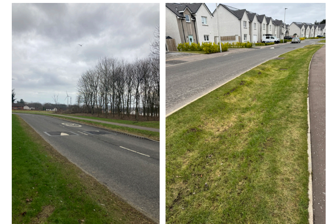
SuDS along the carriageway
