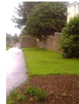
Looking south; note bush at wall - may cause problems in future
