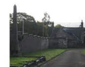
Grass verge at south east of cemetery near hearse house Potential for use for additional cremated remains plots. Also potential refurbishment of hearse house
