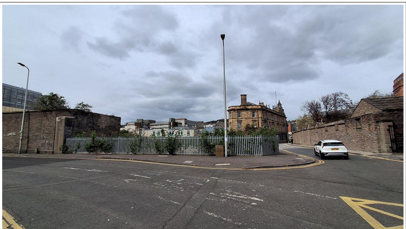
Figure 4: View of Site From Willison Street
