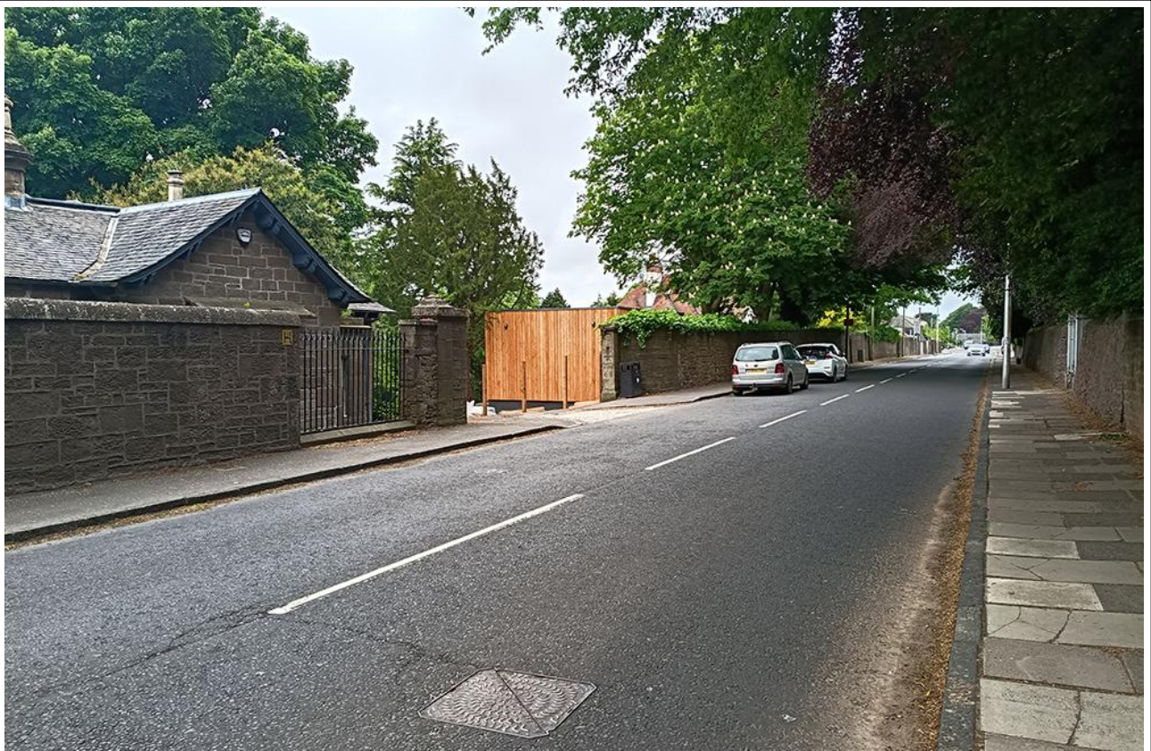
Figure 3 – Perth Road Looking West to Shared Access
