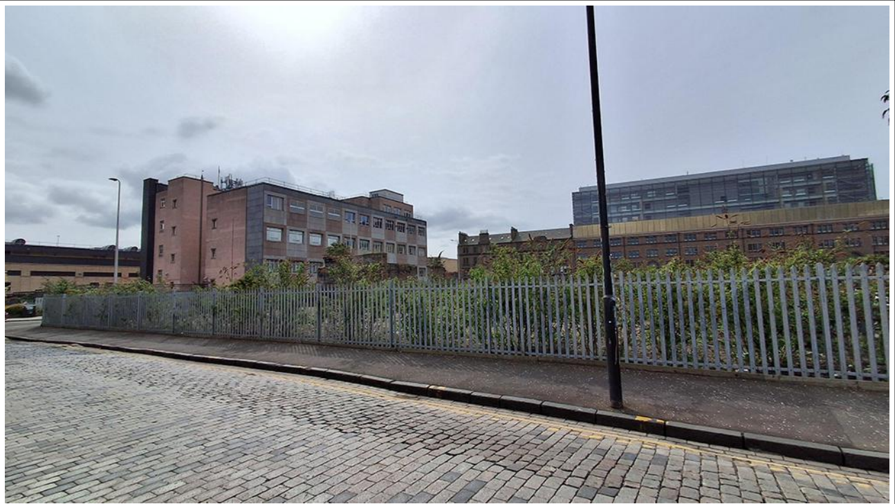
Figure 3: View of Site From Barrack Street
