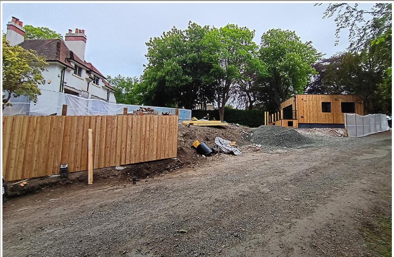
Figure 5 – Garden Building from the Shared Access
