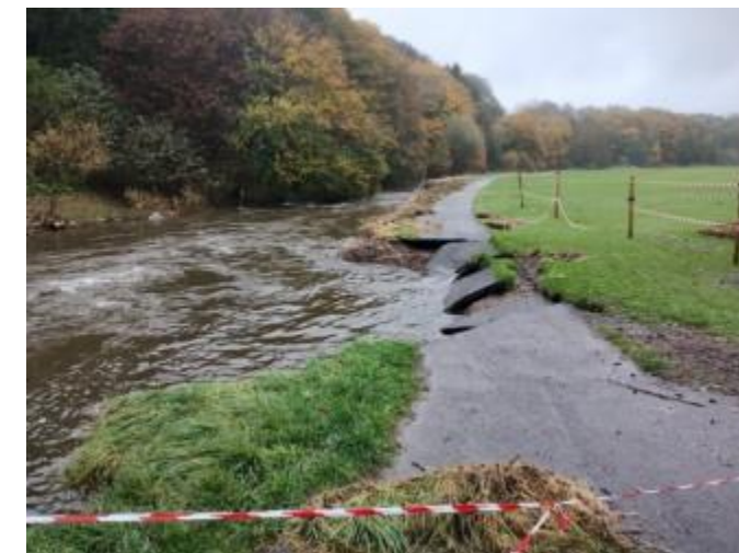
Figure 17. Storm damage to Finalthen Park, where paths were washed away in 2024, Source: Dundee City Council
