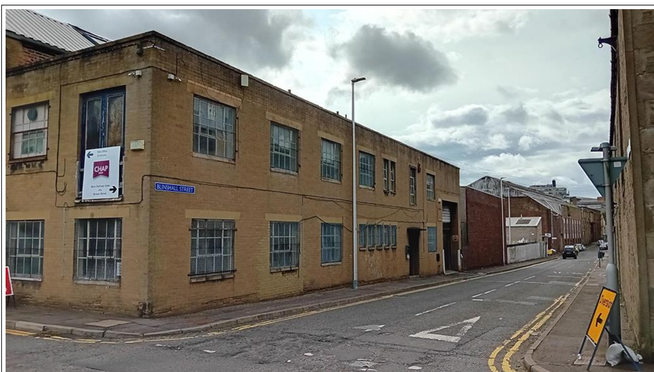
Figure 6 – View of Site From Blinshall Street
