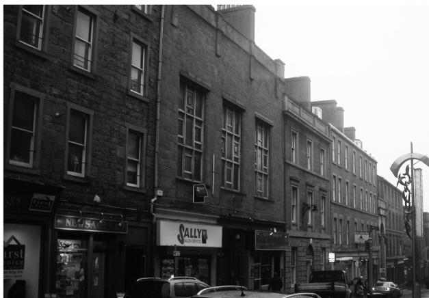
by cast-iron cluster columns. Delineating the ground and first floor and existing today is a full width moulded cornice and band course. There was also a coped parapet with stepped angle dies and four pendant dies. The original stepped angle dies have been filled in to form an extended string course above the coped parapet of the building. The pendant dies have also been removed.
