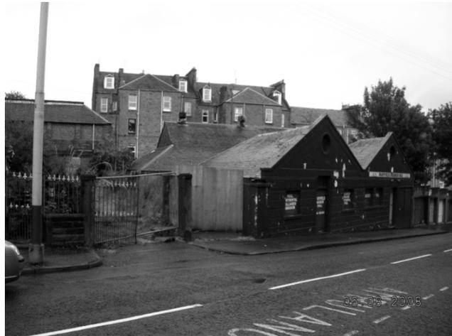
The site itself has a stone frontage with engineer brick north, south and eastern elevations. There are ornate bull's-eye windows in the front elevation with the slate roof being dual pitched with a trough gutter running along the margin
