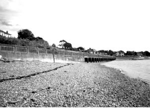
The existing concrete clad iron structure is showing signs of significant erosion with rust from the iron skeletal structure staining the concrete superstructure of the elevated walkway.
