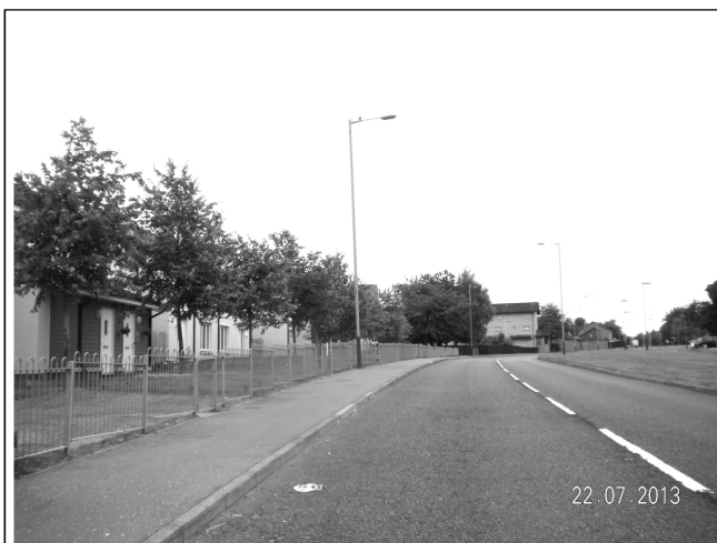
Figure 4 – Longhaugh Road Looking North
