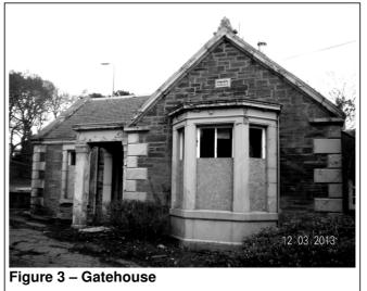
Armitstead House (see Figure 3). The property is currently unused and appears to have been this way for several years. The building itself is showing significant signs of distress generally from wear and tear and misuse, however, there are additional signs of damage due to water penetration. This has further been exacerbated from what appears to be a lack of maintenance of the property in recent years.
