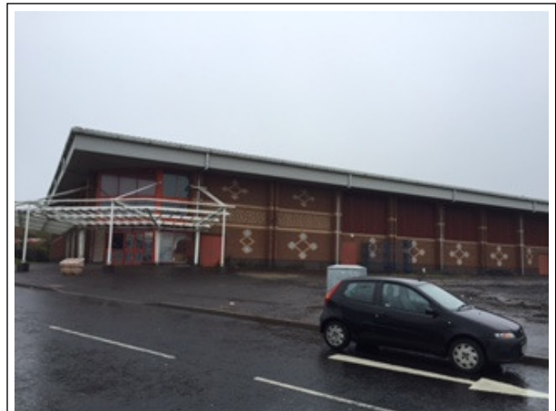
Figure 1 – Photograph of Former Night Club Building
