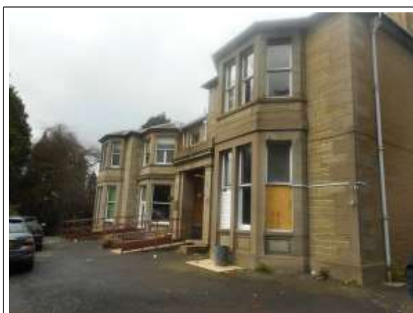
Figure 1 – Anton House – Front Elevation
