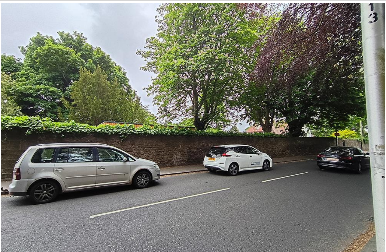
Figure 4 – View From Perth Road
