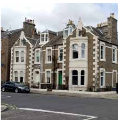
Traditional Stone Built Property
