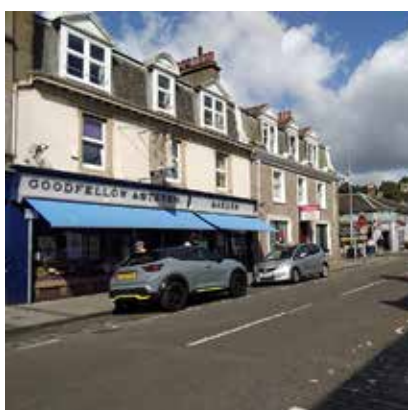
Traditional Shop Fronts
