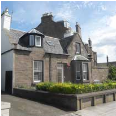
Traditional Stone Built Property
