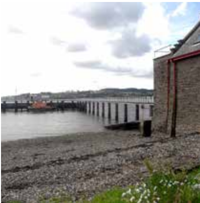
Broughty Ferry Lifeboat Station and pier extension
