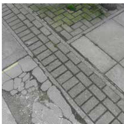
Mix of materials used in footway treatments
