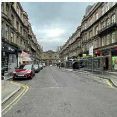
High Quality Paving on Whitehall Street
