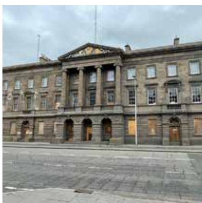
Former Customs House & Harbour Chambers Building
