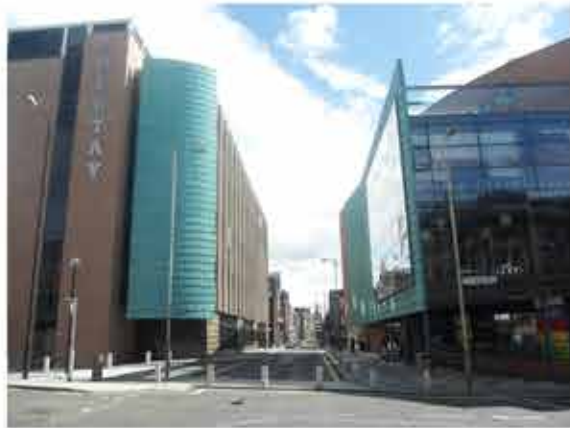
Above - View East along Bell Street
