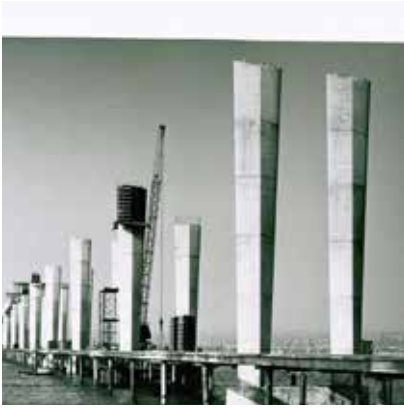
Tay Road Bridge Construction
