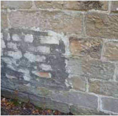
Insensitive wall repair
