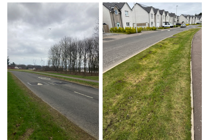
SuDS along the carriageway
