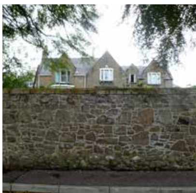
High stone boundary walls
