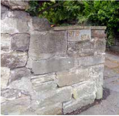
Existing Boundary Wall
