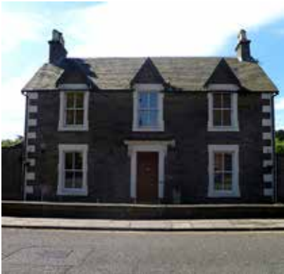
Traditional Property within the Conservation Area
