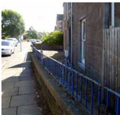
Boundary wall and railings
