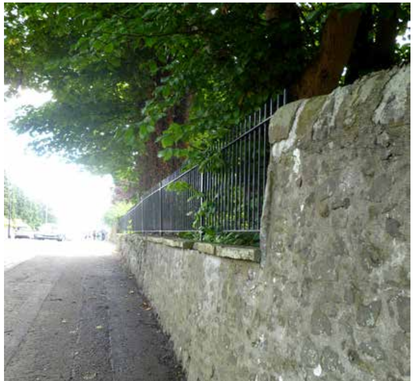
Boundary walls and mature trees
