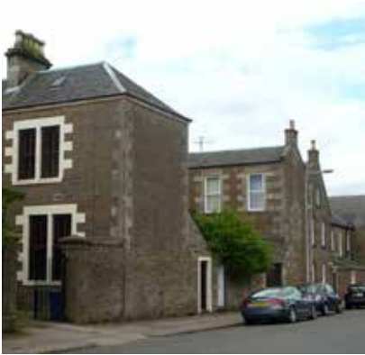
Houses along Camperdown Street
