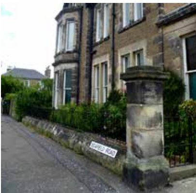
Existing stone gatepier and walls
