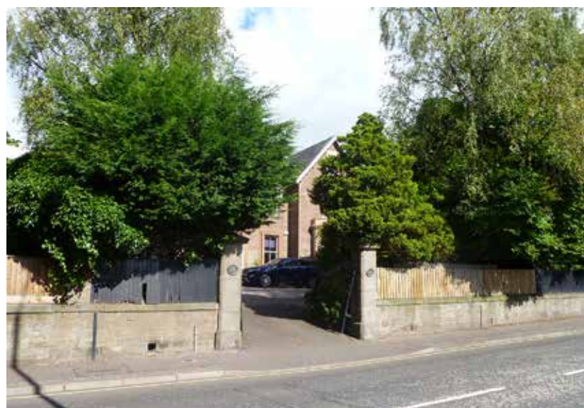
Boundary railings replaced with timber
