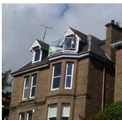
Traditional dormer windows and modern balcony
