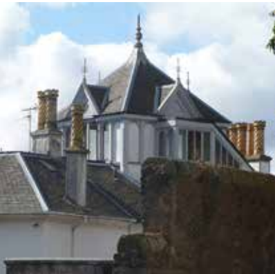
Roof detail and chimneys
