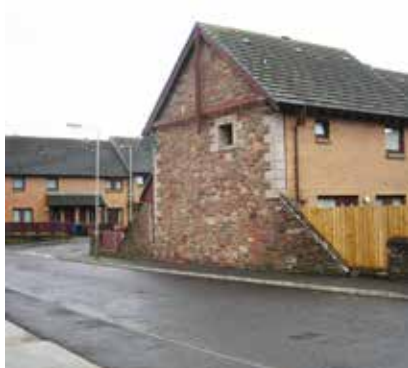
Re-Use Of Materials
