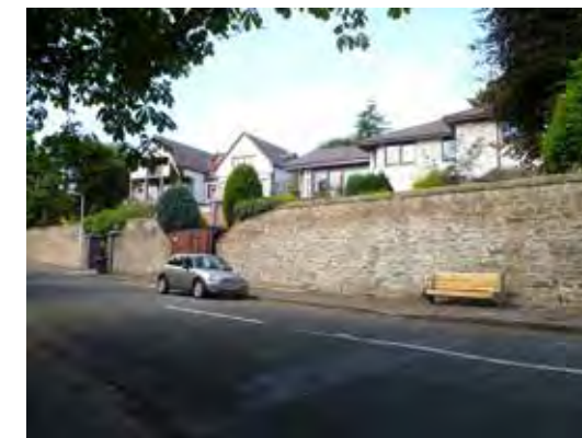
High boundary walls of Bughties Road
