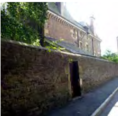
Stone boundary walls
