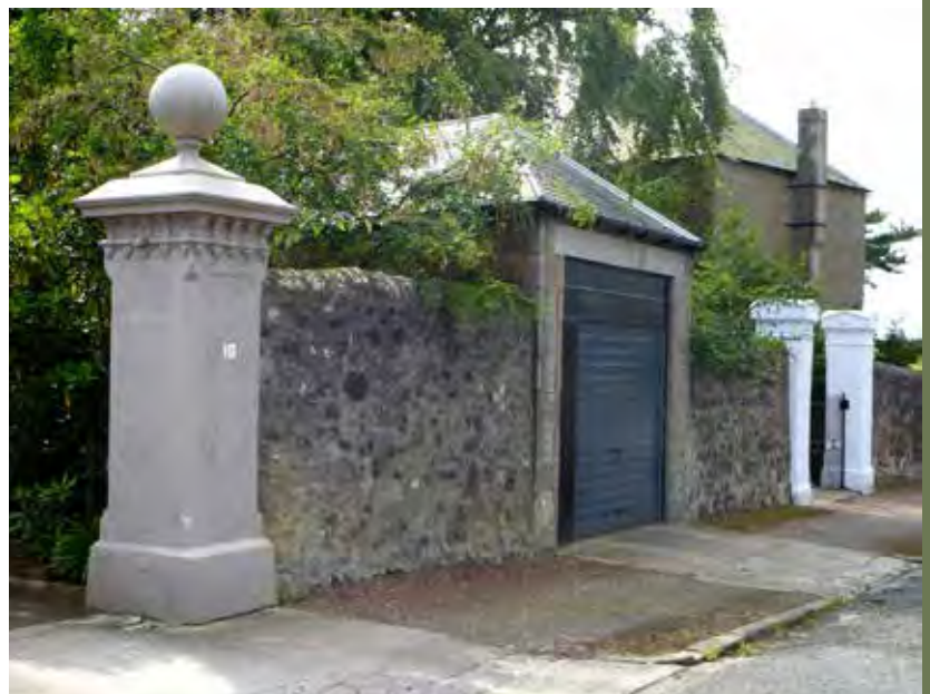
Traditional gatepiers and walls
