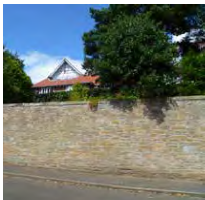
Stone boundary Wall
