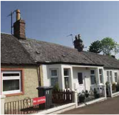
Modern replacement windows
