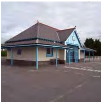
Toilet Facilities at Mill St
