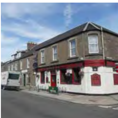
Public House with Satellite Dish on Prominent Elevation
