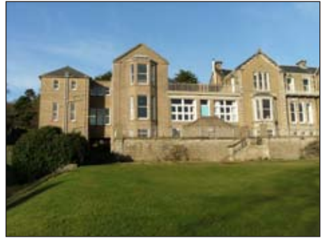
The West wing may be demolished
