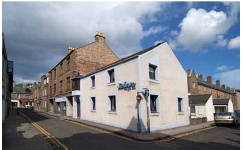
Union St, view towards Brook St
