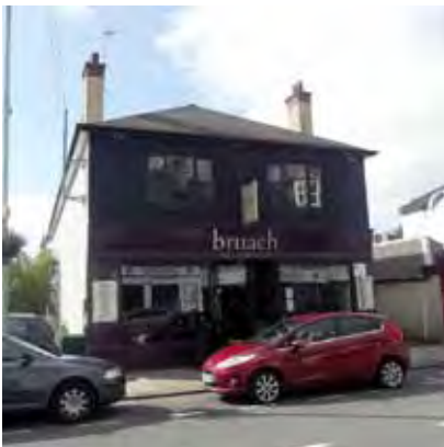
Restaurant along Brook St
