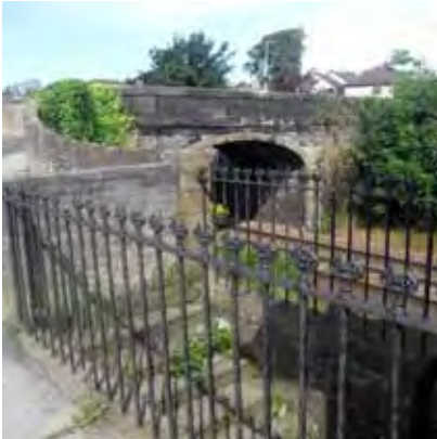
Bridge over railway line through Broughty Ferry
