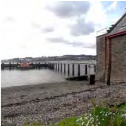
Broughty Ferry Lifeboat Station and pier extension
