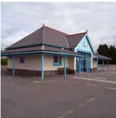
Toilet Facilities at Mill St
