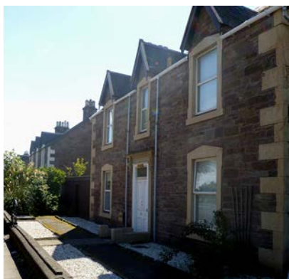
Painted quoins and boundary walls
