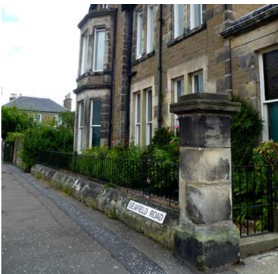
Existing stone gatepier and walls
