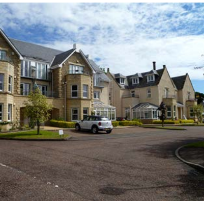
New housing at Bader Square
