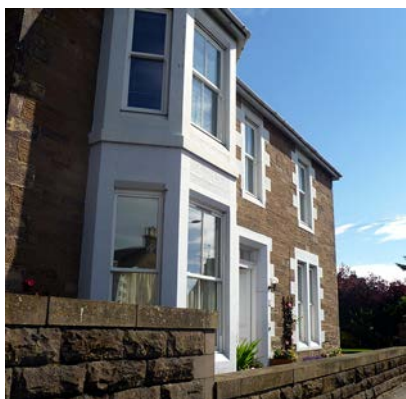
Bay windows and boundary walls
