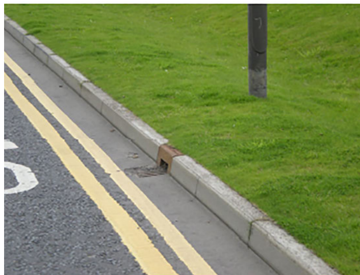
Figure 12: Examples of some roadside SUDS details. Source: SUDS For Roads (SEPA)
