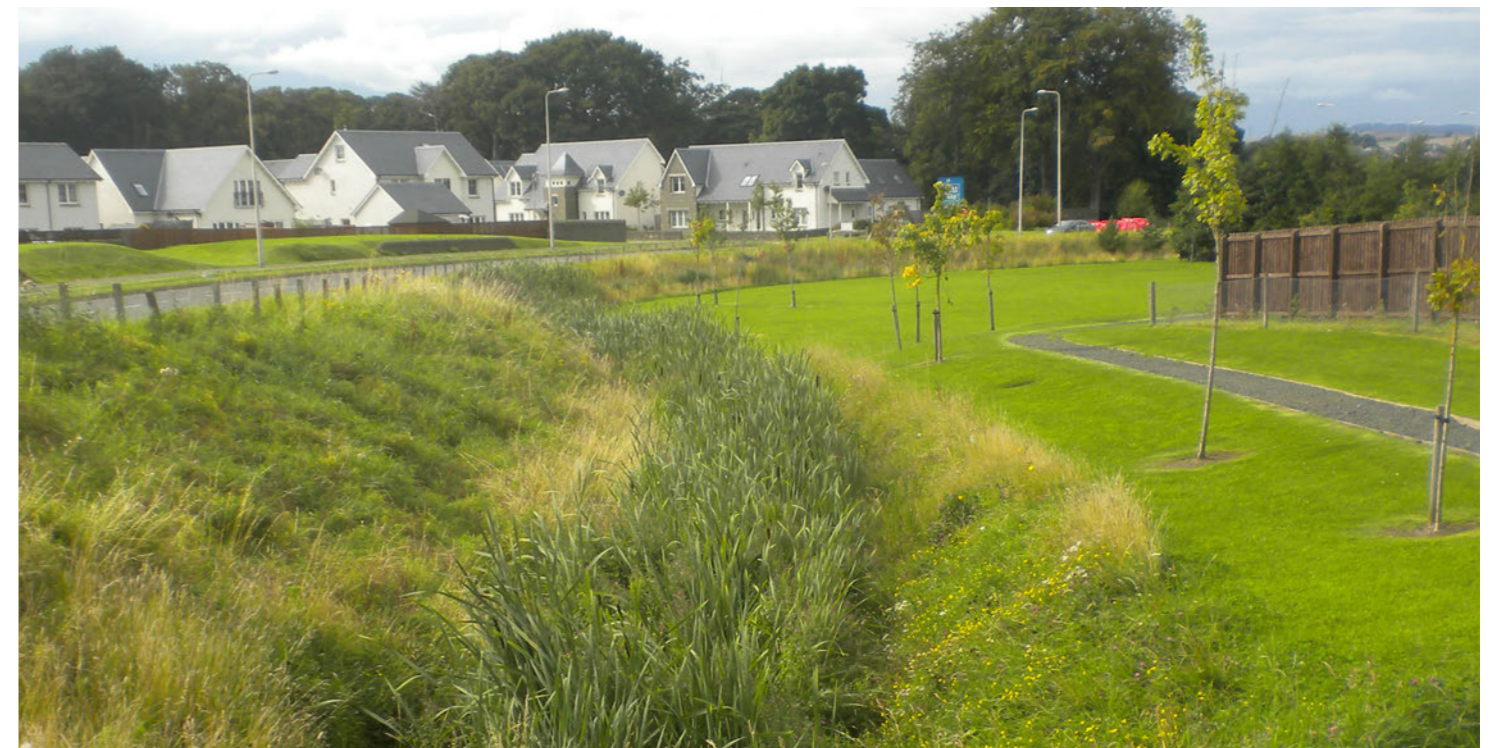
Figure 02: Examples of SUDS throughout the city (Top: Baldrigon, Bottom: Clearwater)
