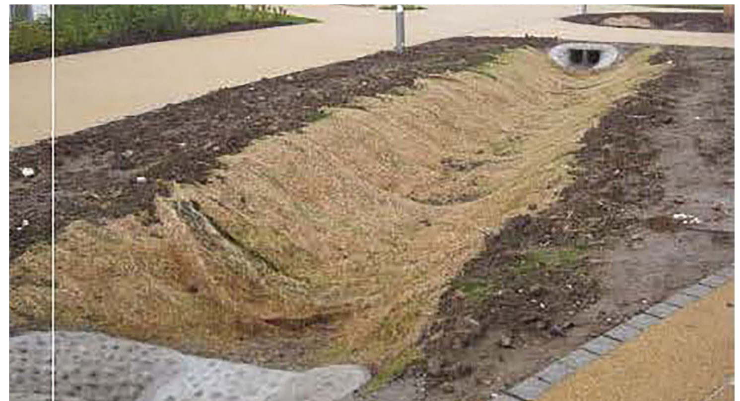
Figure 17: A swale under construction. Source: The SUDS Manual C753 (2015)
