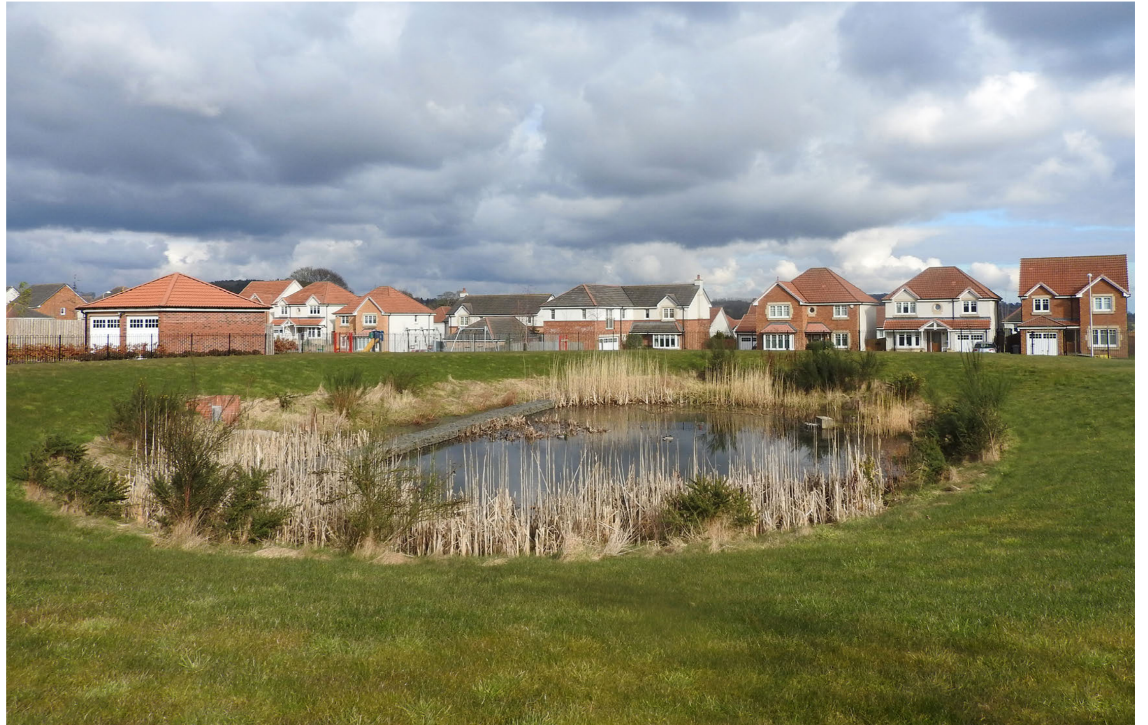
Figure 18: View towards the Baldragon Pond.
